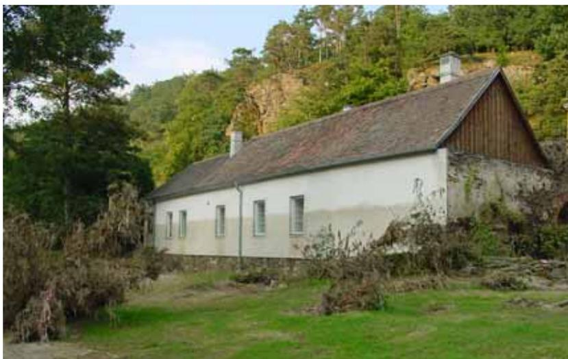
**Fig. 2** Flood marks of the August 2002 flood at the bank of the Kamp near Rosenberg (Reach 5). The peak flow was about 570 m<sup>3</sup>/s. Photo courtesy of Pfarre Horn.
